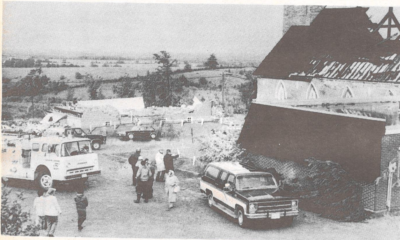
St. John's Church in Ida, built in 1867, suffered extensive damage in the severe storm. Crews assess the repairs required.
