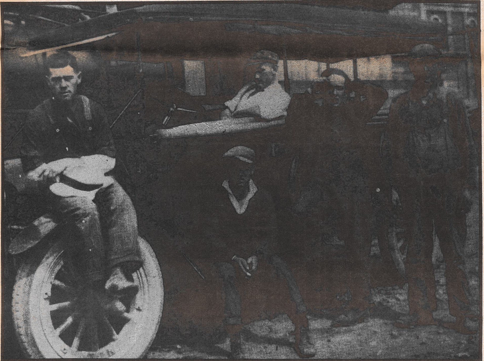
Moving the hydro poles in the Twenties
